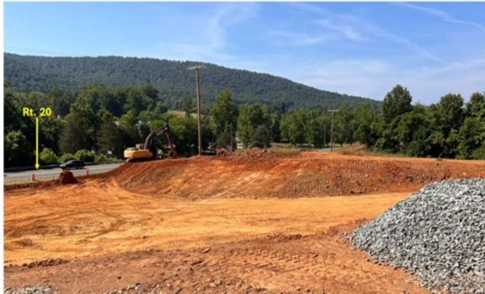
Biscuit Run Park Phase 1a Entrance Excavation
